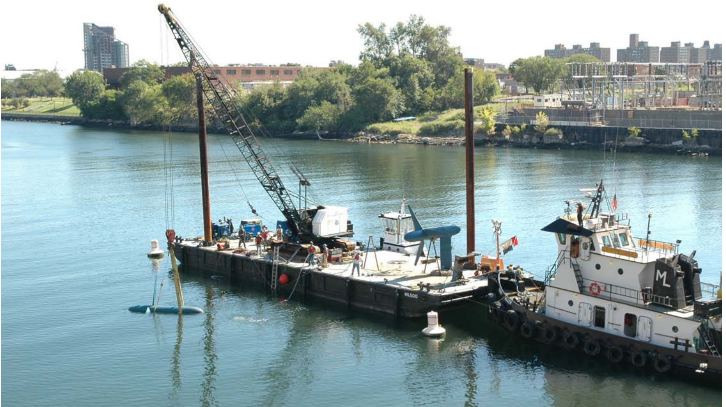
Free Flow System turbine installation in the East River, 2008.
